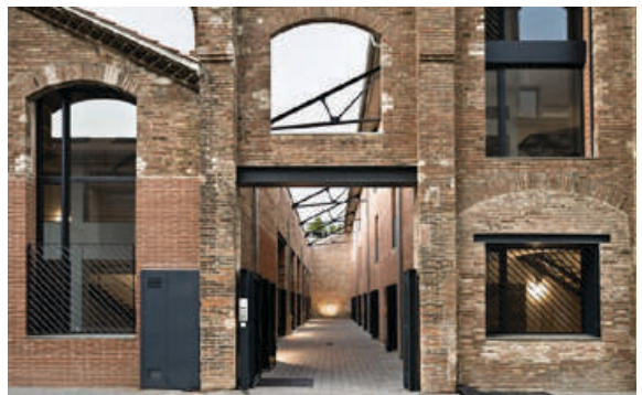
GARCÉS DE SETA BONET, Transformation of an ancient distillery into housing and working spaces, Poblenou, Barcelona, 2009
